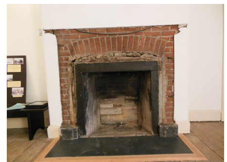
The mantel being removed for restoration, revealing further historical evidence; photographs courtesy Carolyn Gamble.
